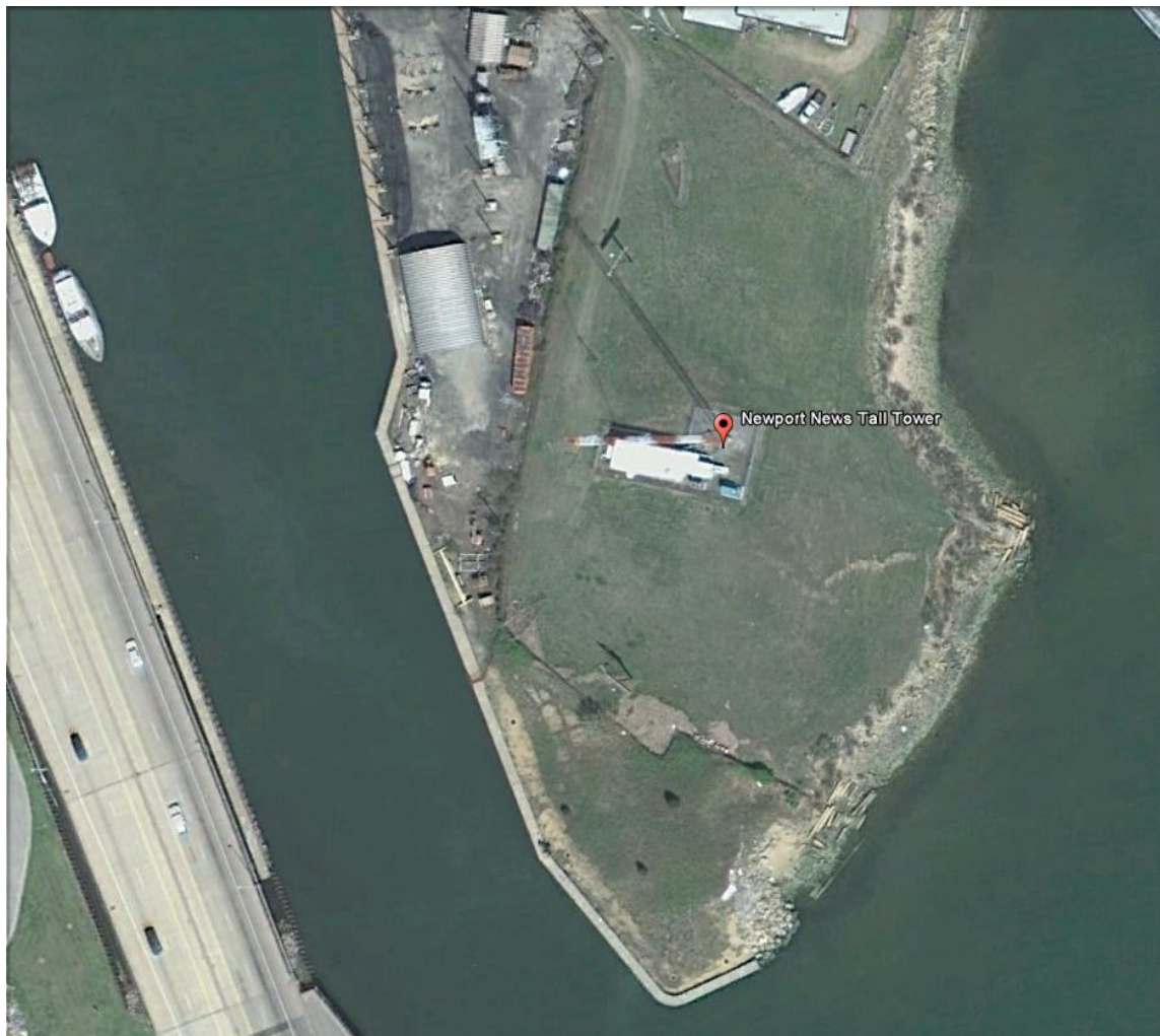
Figure 1: Close-up Google satellite image of the tower.
